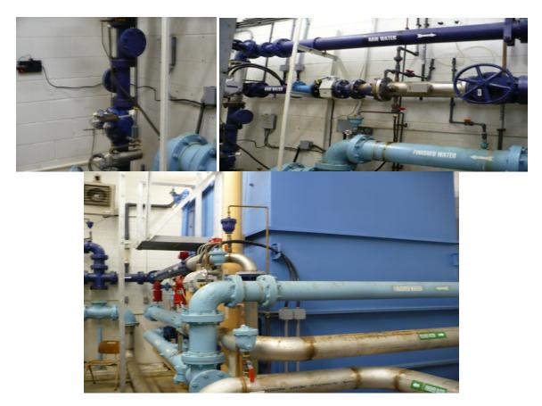
Primary disinfection is provided using sodium hypochlorite and ultraviolet light. Secondary disinfection is being provided using stabilized hydrogen peroxide. The peroxide is injected prior to the clearwells and a residual is maintained through the distribution system.
