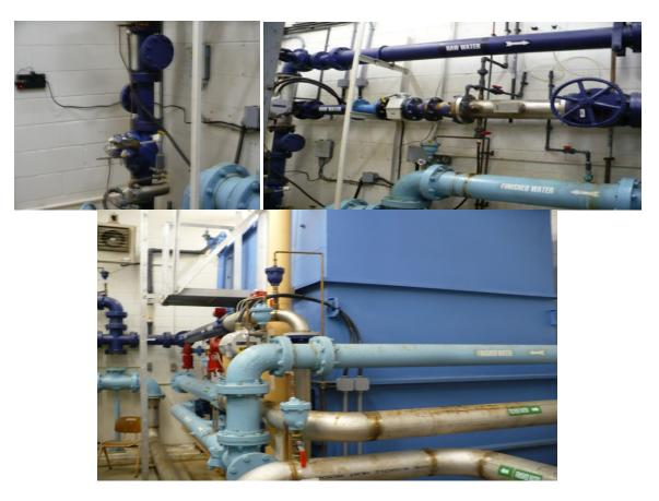
Primary disinfection is provided using sodium hypochlorite and ultraviolet light. Secondary disinfection is being provided using stabilized hydrogen peroxide. The peroxide is injected prior to the clearwells and a residual is maintained through the distribution system.
